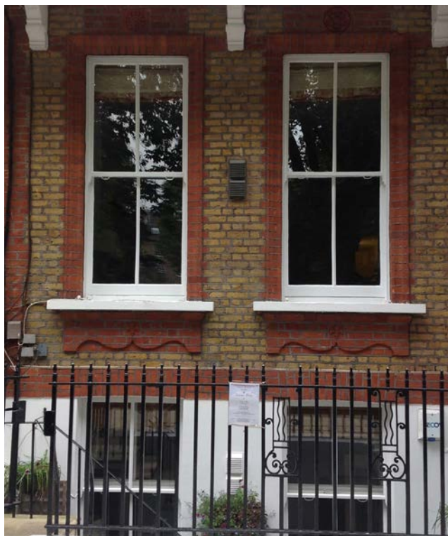
Domestic Revival sashes with single glazing bar
