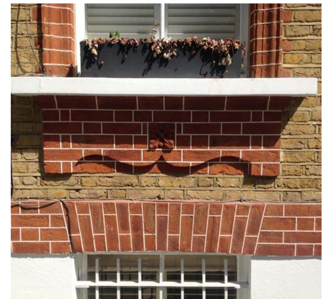
Tuck pointing and fine lime pointing
