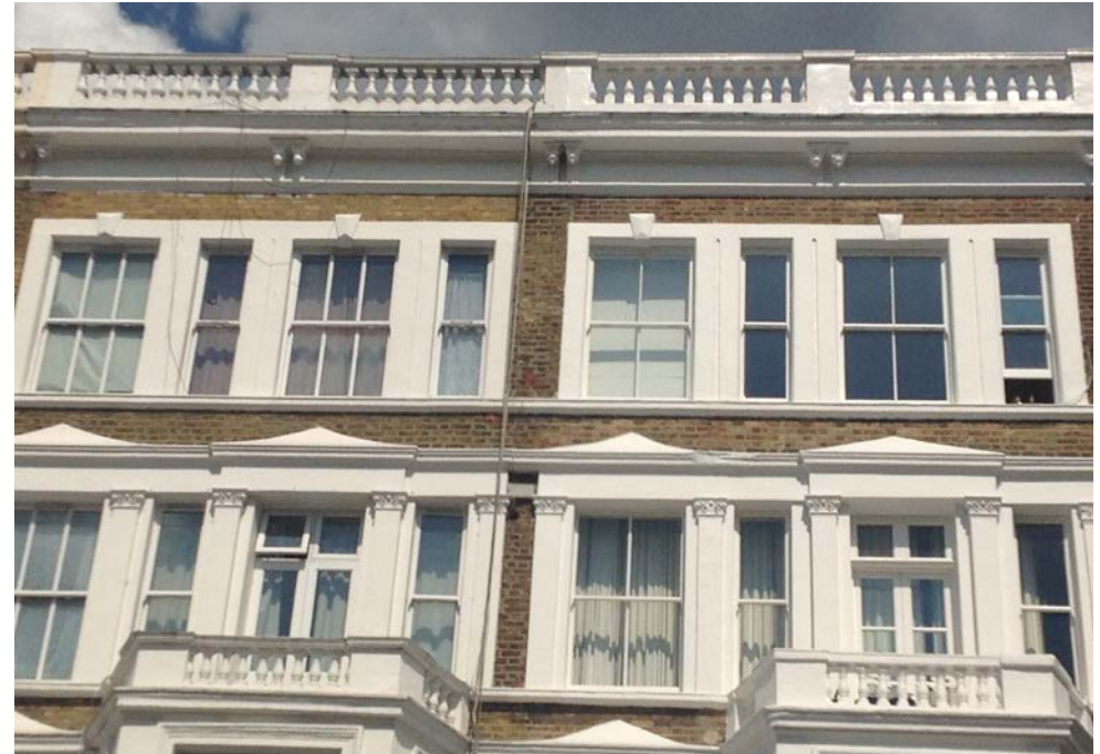
Classically inspired parapet with balustrade and bracketed cornice, Nevern Road
